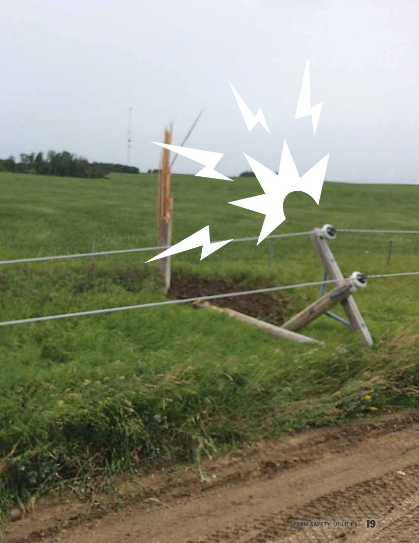
If you are in a vehicle, tractor, or other large piece of equipment and it hits a power line, the driver can try to break the connection by moving the vehicle or machinery away.
