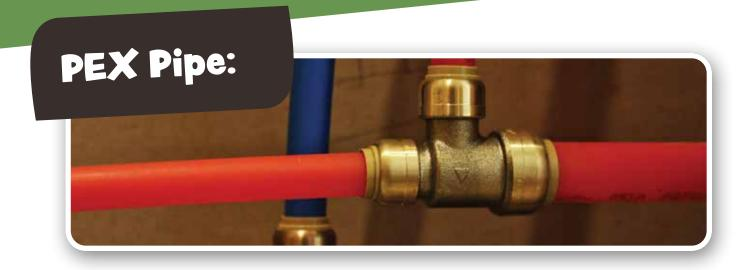
PEX Pipes (or cross-linked polyethylene pipes) are one of the newest and most popular types of water pipes. PEX is tough enough to withstand water pressure but is also flexible enough to weave throughout walls, ceilings, basements, and crawlspaces, delivering water to our homes and businesses.<sup>15</sup>
