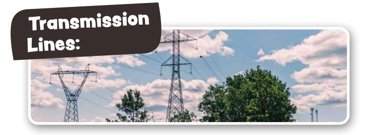
Transmission lines are high-power-level lines connected right to the power substation that transmits the electricity. Transmission lines are above the ground and attached to steel towers or high poles. They can carry up to 800,000 volts, so the electricity can travel long distances without losing its power. There are also some underground transmission lines, but these are less common.<sup>13</sup>
