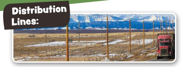
Distribution lines are medium-voltage-level lines that run in the country and through communities. Their voltage can be between 2,000–25,000 volts, with lines mainly occurring underground in cities and above ground (held up by poles) in rural communities like farms and acreages.<sup>13</sup>
